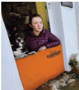
Installing temporary barriers across exterior doors and windows can help keep floodwater from entering a home.
