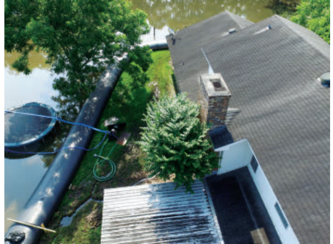
A perimeter of water-inflated barriers protected a house from flooding during a season of record-setting rainfall in Rosharon, Texas, in 2016.
