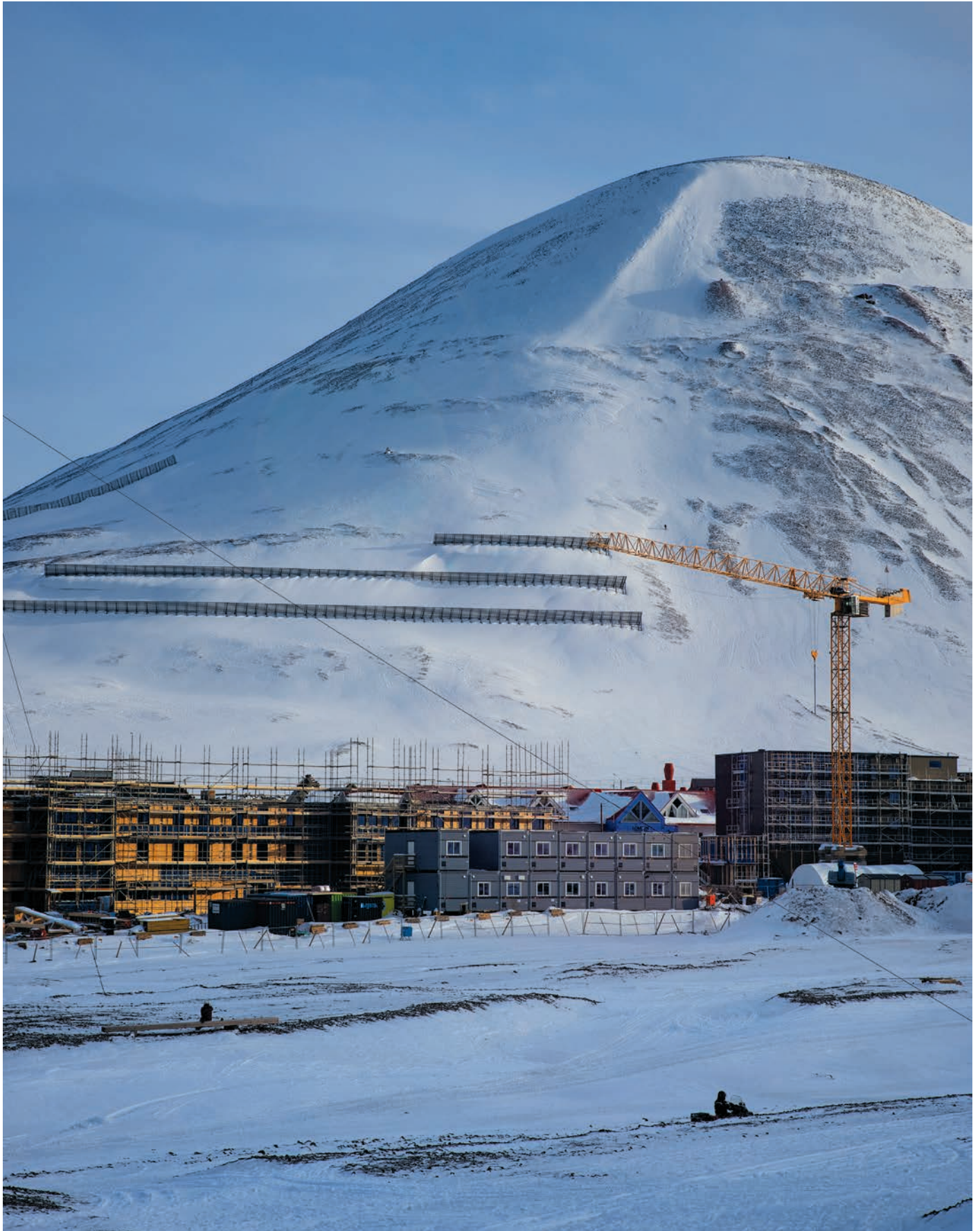
HIGH-DENSITY HOUSING and university dormitories are being built in anticipation of more jobs and greater workforce turnover. Steel fences (seen on mountainside) have been installed to thwart avalanches.
